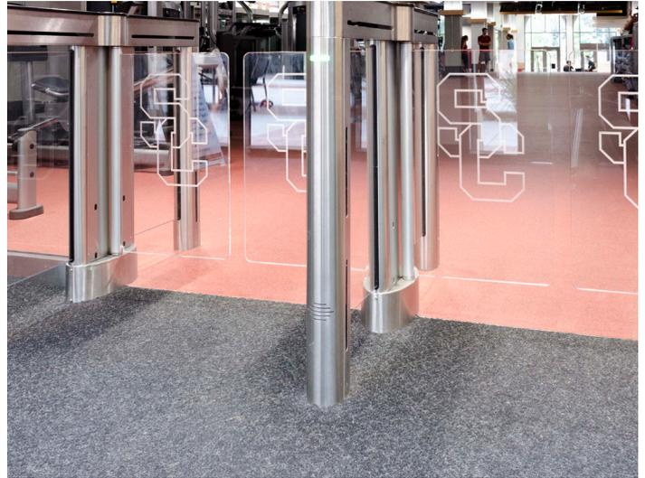
For the cardio and functional training areas, Gilman selected Ecore Performance Rally flooring. This 14.5mm product combines a 2.5mm wear layer with a 12mm shock-absorbing base layer and is engineered to absorb the impact force related to aggressive functional training.
